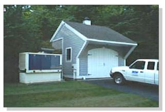
Village at Highland Park is located in Hopkinton, MA and draws its water from two underground wells located near the pump station. The water is stored in an 8000 gallon atmospheric storage tank at the pump station and two booster pumps send it uphill to the 200 gallon hydropneumatics tank that supplies pressure to the distribution system.
