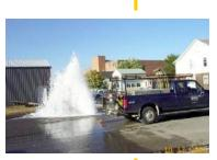
Backsiphonage may occur due to a water main break or other lowpressure incident such as a fire.
